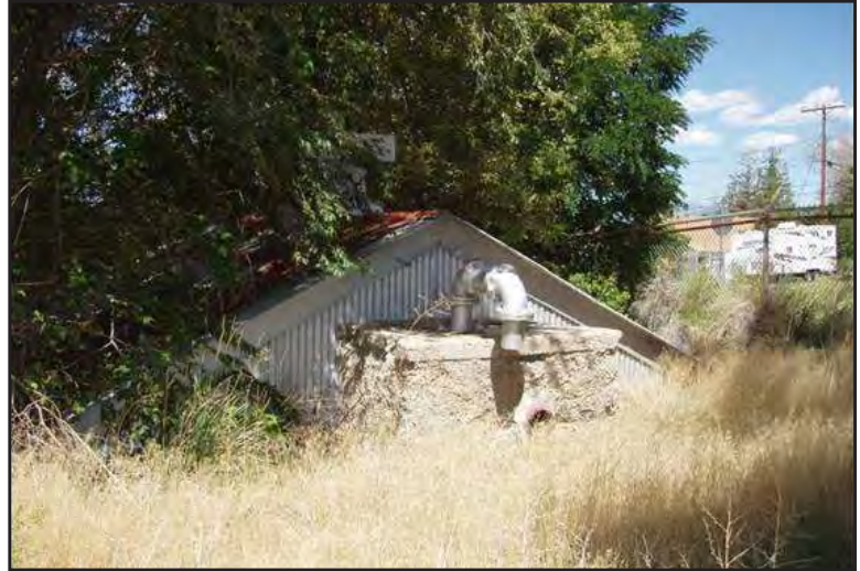
Wellhead in Mc-Gill-Ruth.
