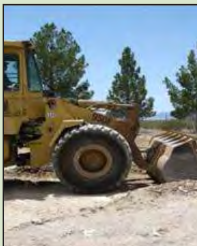
NWRPO Laydown Yard remediation activities. Source: BEC files.
