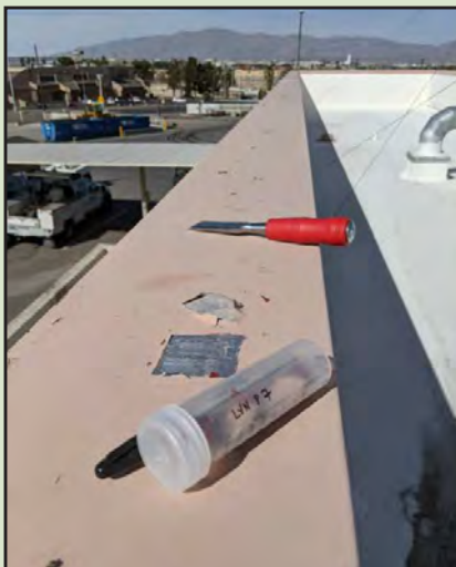
Photo of lead-based paint sampling being conducted at the North Las Vegas NDOT facility.
