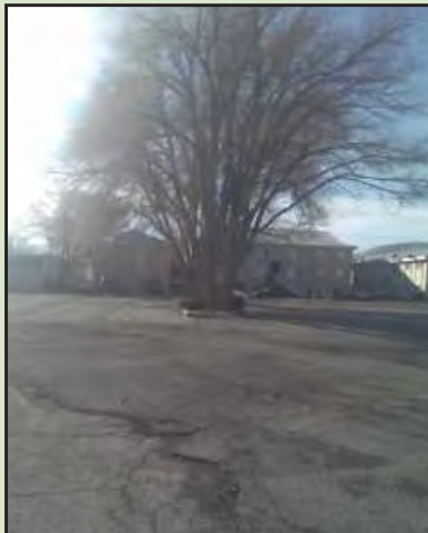
Southern parking area and concrete-lined plant area.
