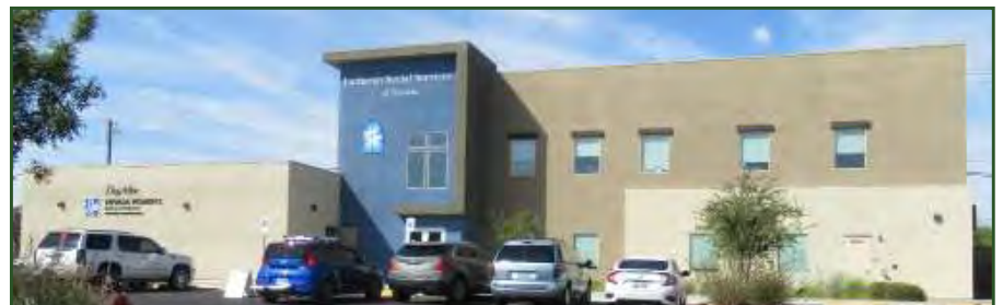
East elevation of the Journey Senior Services Center Source: BEC Files
