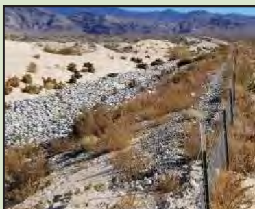
Additional drainage channel. Source: BEC files.
