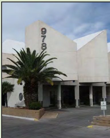
Apartment building front. Source: BEC files.
