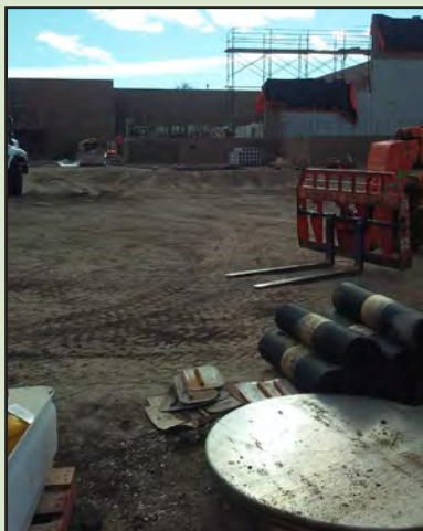
Detention Center, North Side, Churchill County, Nevada. Source: BEC files.
