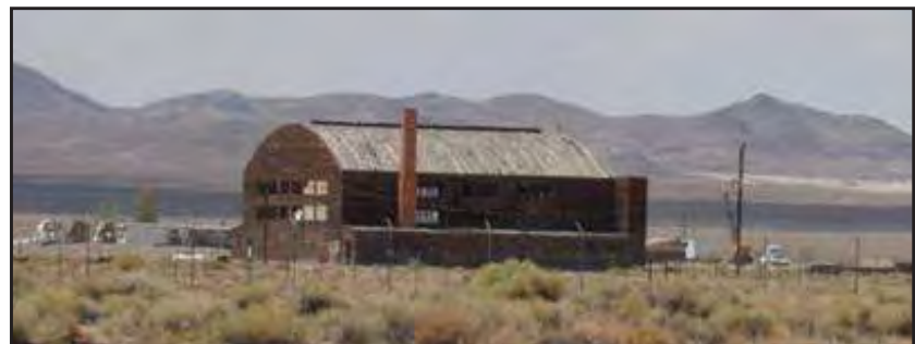
Tonopah Airport hanger. Source: BEC files.
