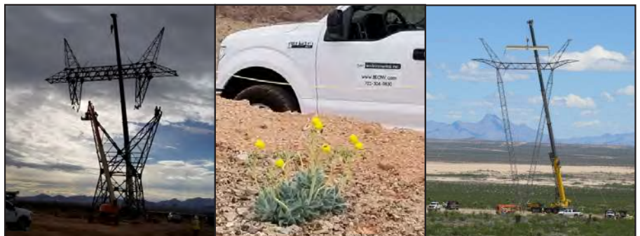
Site construction activities. Source: BEC files.
