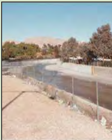
Clark County flood control facility. Source: BEC files.
