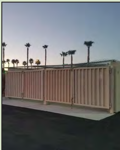
Concrete block dumpster enclosure observed on the subject site. Source: BEC files.
