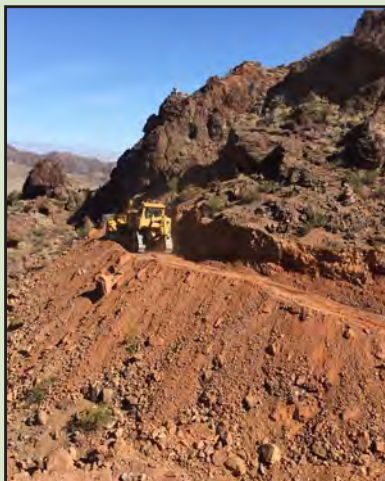
Site construction activities. Source: BEC files.
