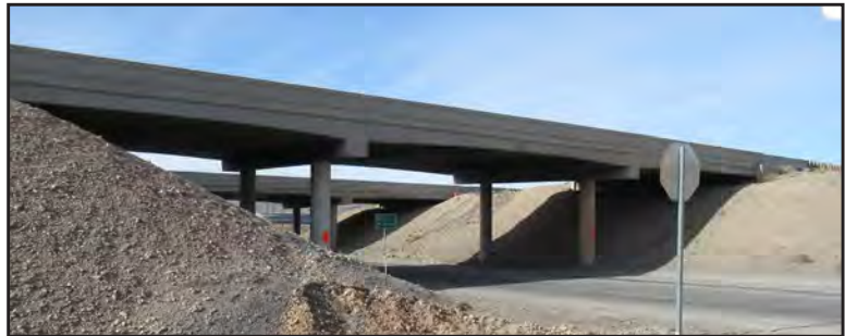
View of bridge in the Garnet Interchange project area.
