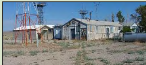
Disturbed areas within and adjacent to the Tonopah Airport FBO building site. Source: BEC files.
