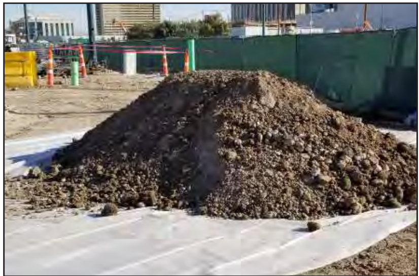
Contaminated soil placed on visqueen for temporary storage pending laboratory analytical results.
