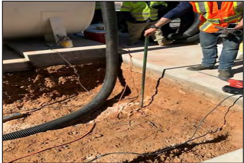
Site cleanup and oversight activities. Source: BEC files.
