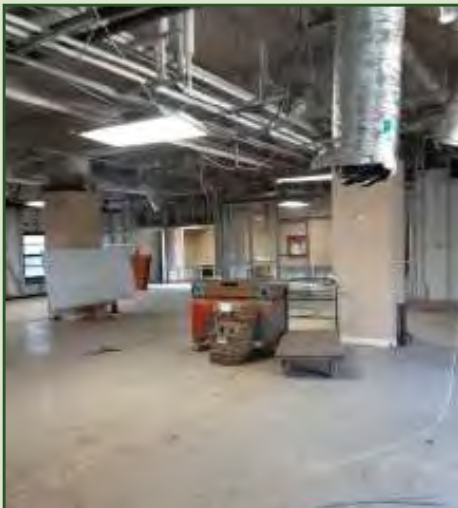
Lobby area undergoing remediation Source: BEC Files
