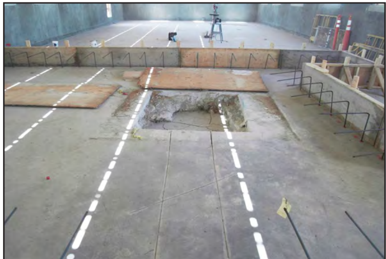
Building 100 soil sampling activities.
