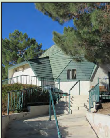
Lakeview Executive Golf Course building. Source: BEC files.
