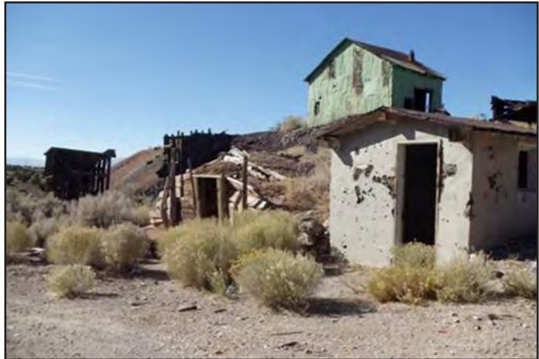
Abandoned mining camp. Source: BEC files.
