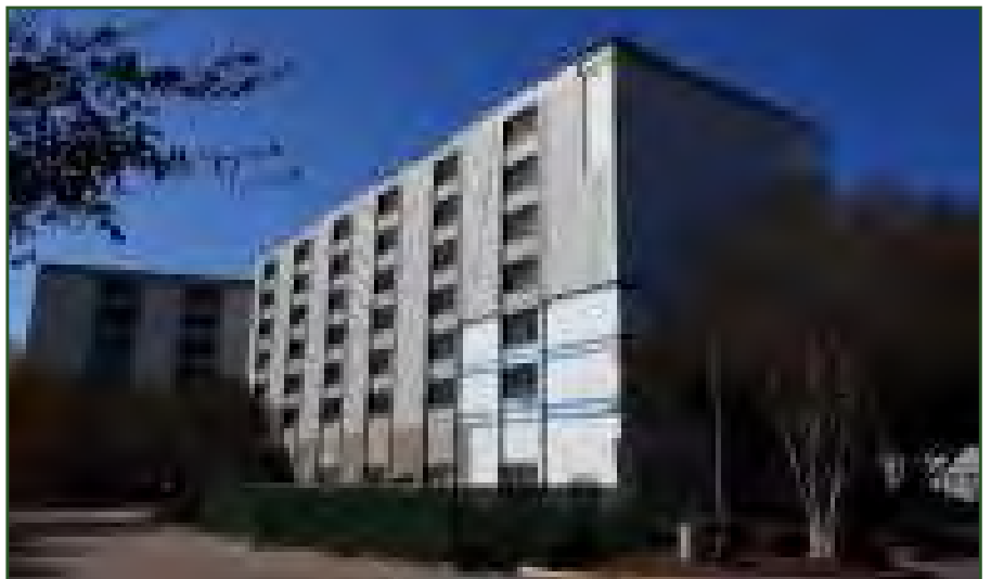
Telephone Road Apartments Source: BEC Files
