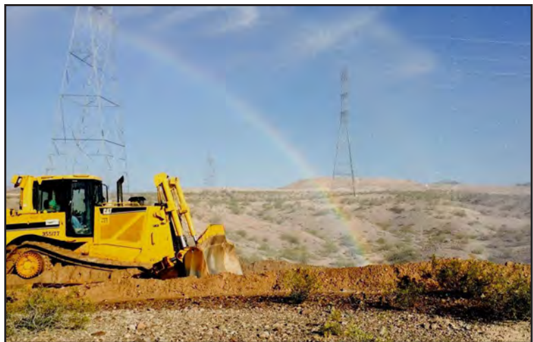
Site construction activities. Source: BEC files.
