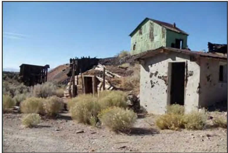
Abandoned mining camp. Source: BEC files.
