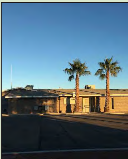
View of SMRYC south elevation. Source: BEC files.
