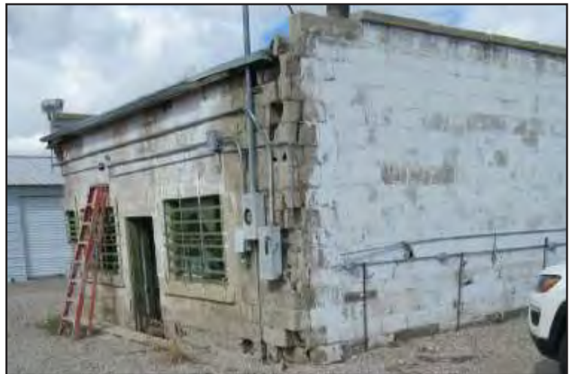
Ely Old Shop Building Exterior Source: BEC files.
