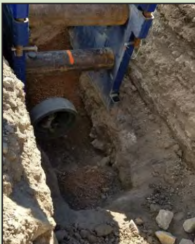
Utility installation in trenches during construction activities Source: BEC files.
