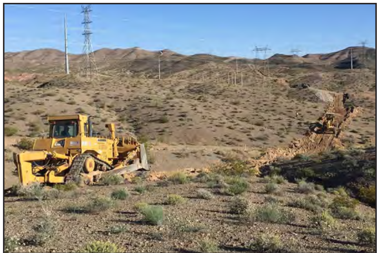
Site construction activities. Source: BEC files.
