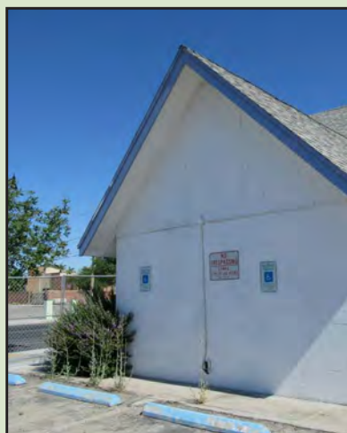
Exterior view of 1100 D Street Source: BEC files.
