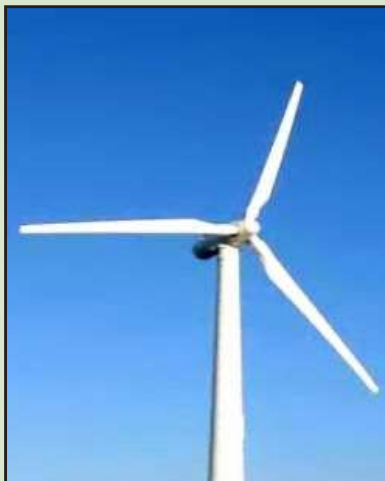
Wind turbine. Source: BEC files.
