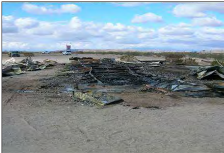
NWRPO Laydown Yard site conditions. Source: BEC files.
