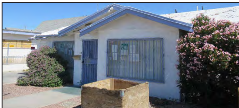
Exterior view of 308 Jefferson Street Source: BEC files.
